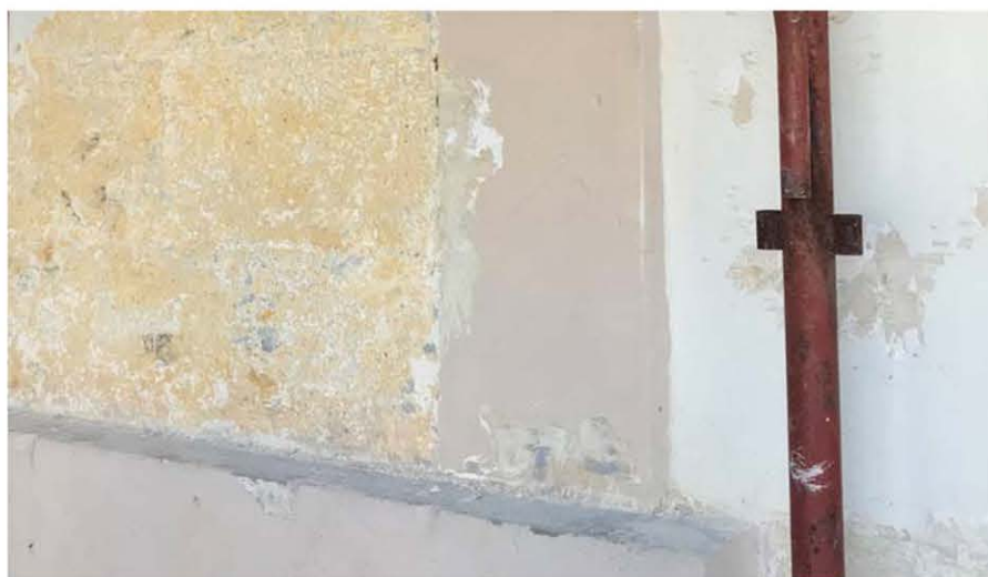
Figure 12: Photo of stratigraphy of paint layers of blocked-up window.
