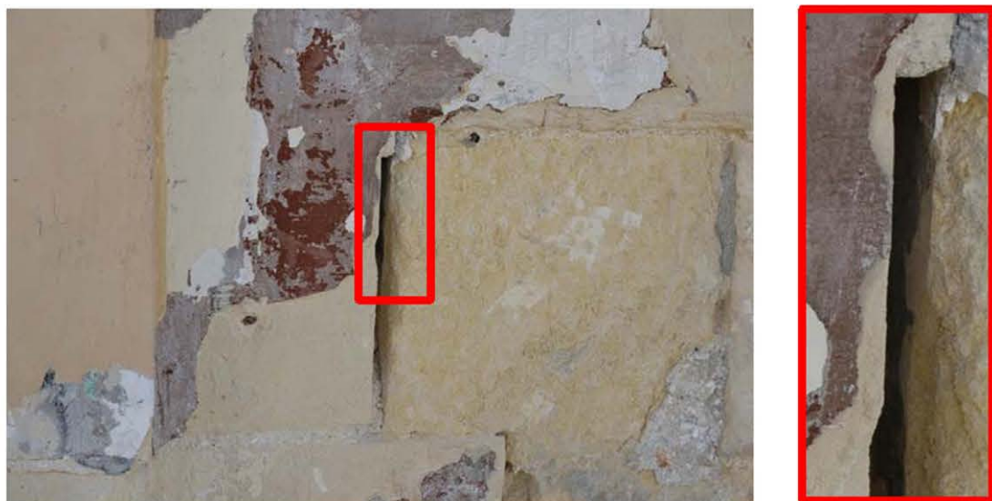
Figure 3: Photo of the exposed construction joint of the extension of the 1882 Station building. Inset photo shows the 1882 Dark (olive) Green oil paint still preserved.
