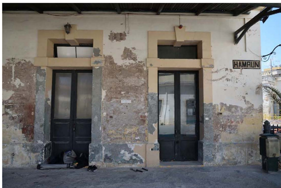
Figure 6: Photo of the Station Building Main Façade with the Earthy Red, Dark (Olive) Green / Dark Cyan (Blue) colour scheme as exposed on site.
