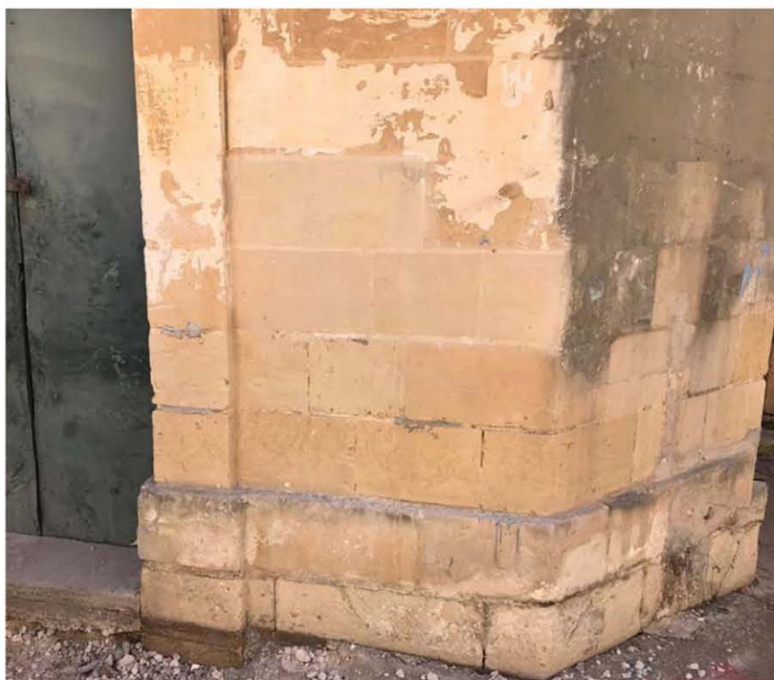
Figure 16: Photo of stratigraphy of paint layers of Pre 1897 Workshop, 1904 Ancillary room
