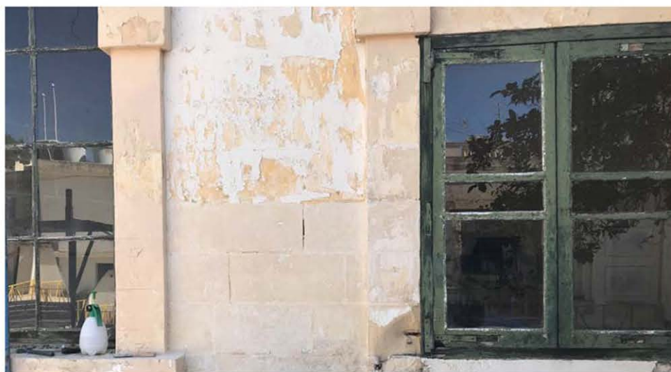
Figure 10: Photo of stratigraphy of external finish of 1904 Station/Workshop North Extension next to the door converted into a window.
