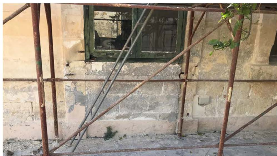
Figure 11: Photo of wall constructed to change the door into window,
