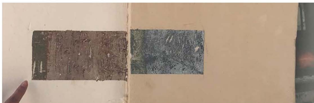
Figure 4: Photo of paint stratigraphy of 1904 extension showing the Dark (Olive) Green Colour as the base colour for the whole façade.
