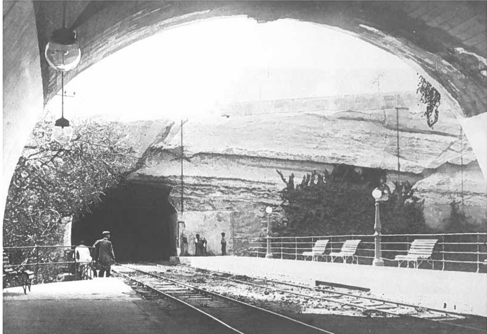
The masonry-lined Valletta Terminus tunnel. The Government improved facilities at the station by putting waiting benches and installing electric lighting. A short viaduct led to the Floriana tunnel which was widened here to enable a longer siding to be laid. In the centre is the water stand pipe for the engines.
