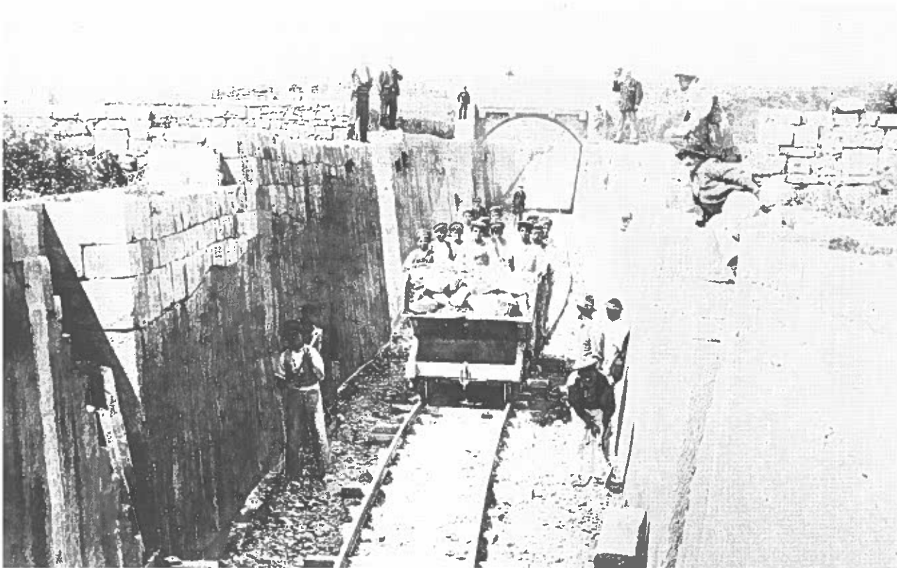
Above: A deep cutting near Tal-Mirakli, Attard. Steps cut in the sides as well as a stone bridge permitted access to fields and roads on both sides of the line. The bridge and the cutting lasted until the late 'Sixties (facing page, top) when both succumbed to extensive housing development Below: The level crossing at the junction of the Mosta-Attard road proved to be one of the most hazardous on the route
